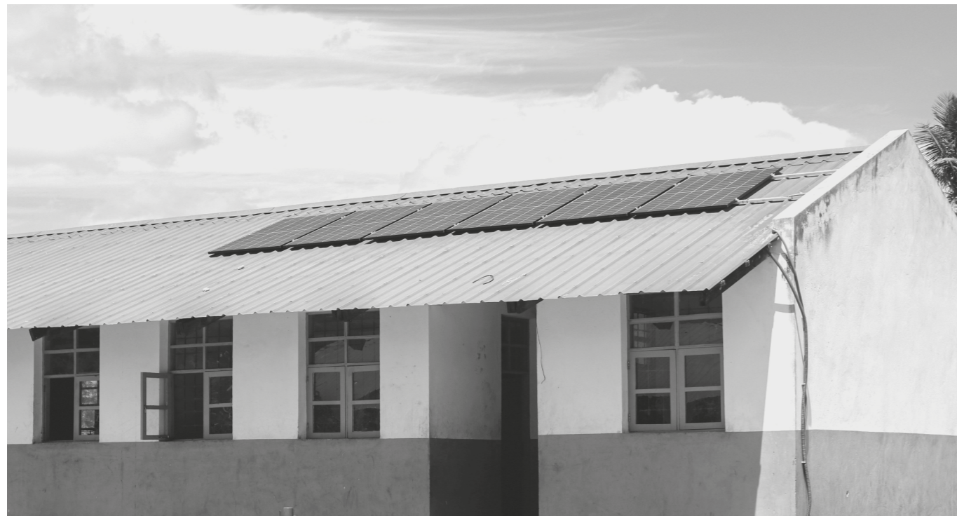
Balama School, Solar PV Installation
